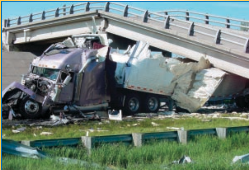
Fortunately for this driver, his truck cab was not directly under the collapsed overpass.
