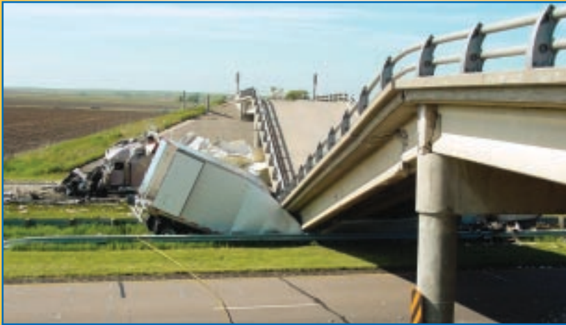
Wreckage of trucks after semi-trailer truck slams into bridge center pier near Big Springs, Nebraska.
