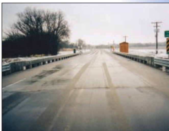
First successful test of melting the snow off the bridge, May 7, 2003.
