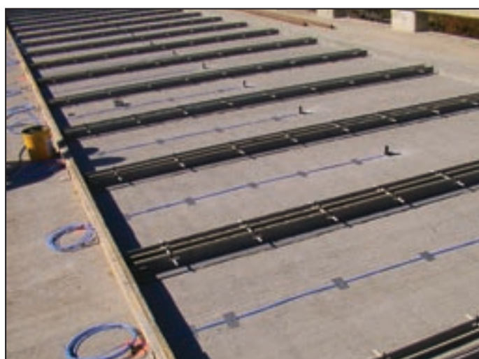
During construction - bridge slabs with cables for electricity.
