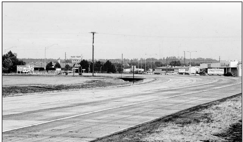
Recently completed section of Highway 20 in Valentine.
