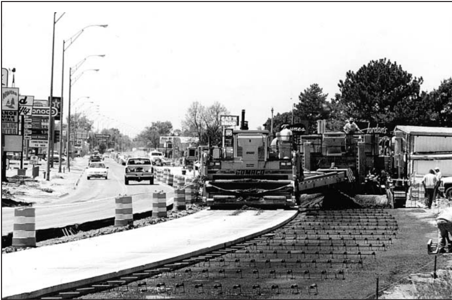
Workers are operating a slip-form paver on Highway 20 in downtown Valentine.
